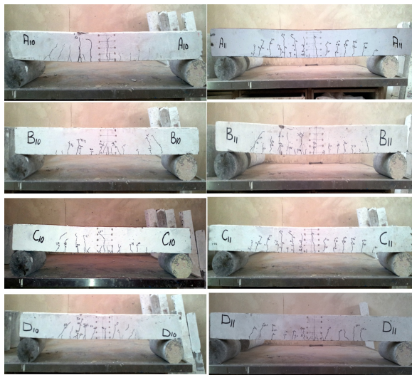
Fig. (9) Crack pattern for tested beams.
